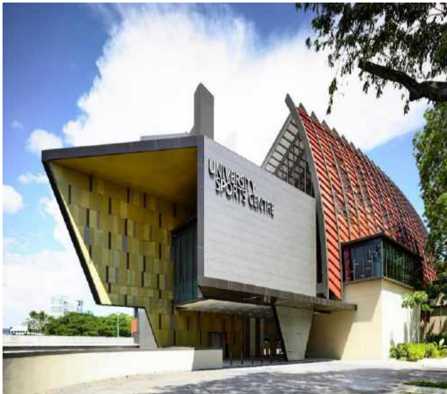
NUS University Sports Centre BCA Construction Excellence Award (Excellence)
